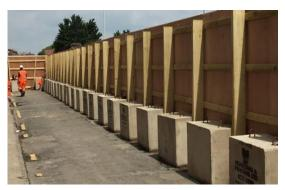
Fig 5.7 Example - Demountable 'Heras' fence and solid timber hoarding with ballast blocks
