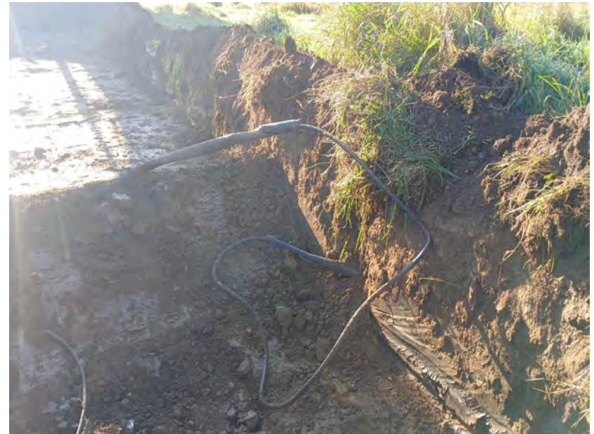
Plate 40: Active water pipe at western end of Trench 28
